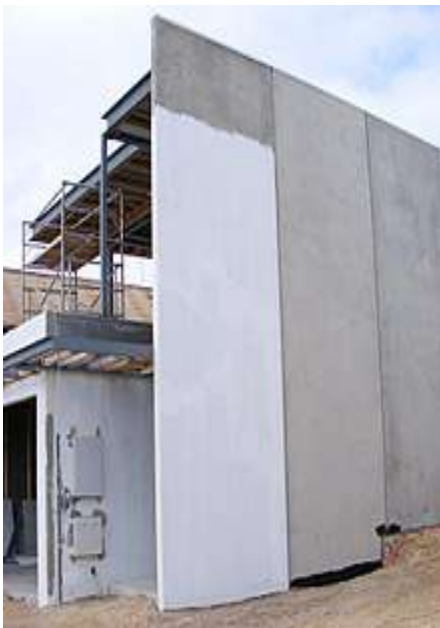
A house being built with prefabricated concrete panels.
