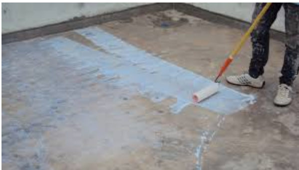
Fig.1. Application of Latex Bonding Agent
