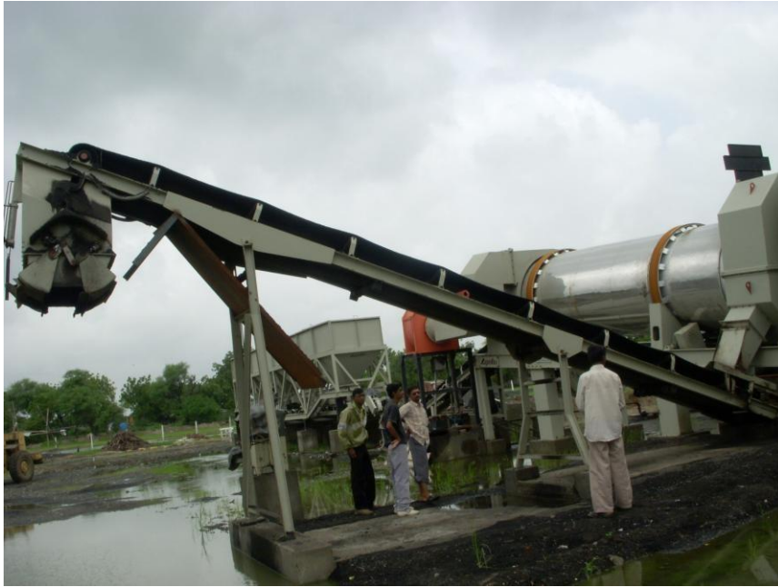
Fig. Load Out Conveyor
