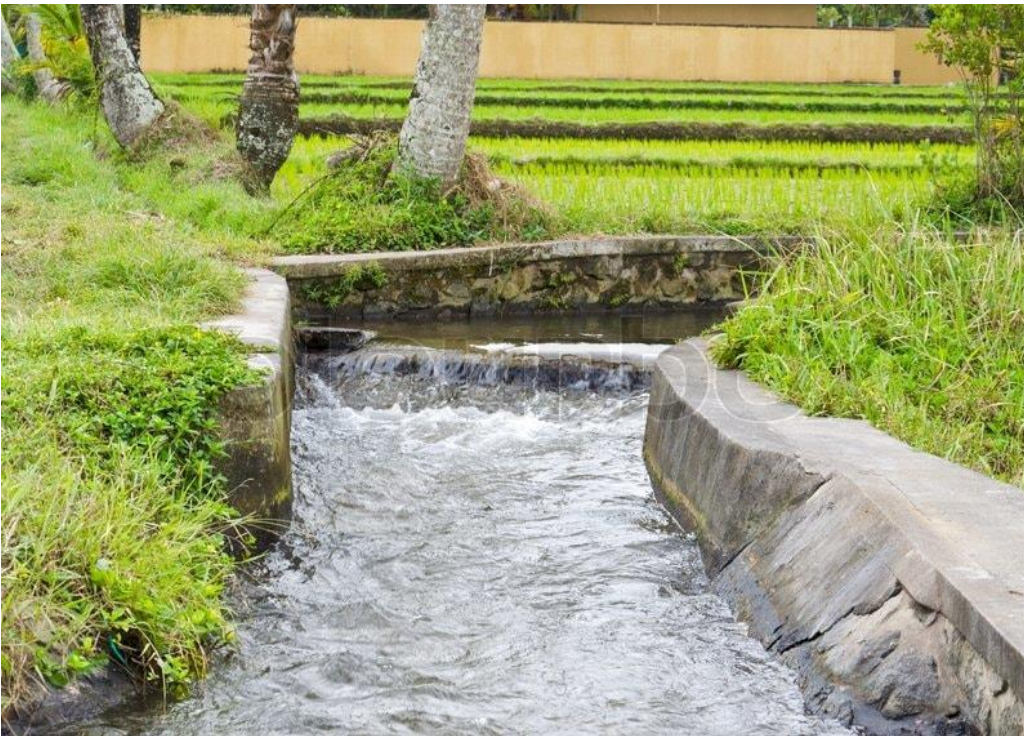
Fig: Irrigation Canal
